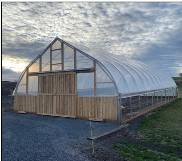
Figure 11. High Tunnel With Wood-Paneled End Walls
