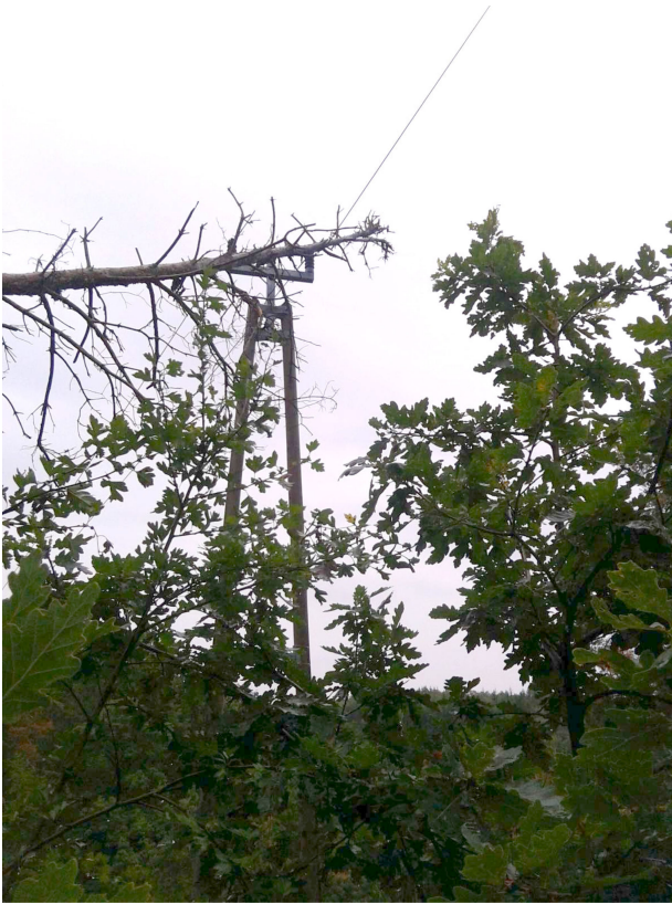
Fig. 1. High impedance fault on medium voltage power line.
