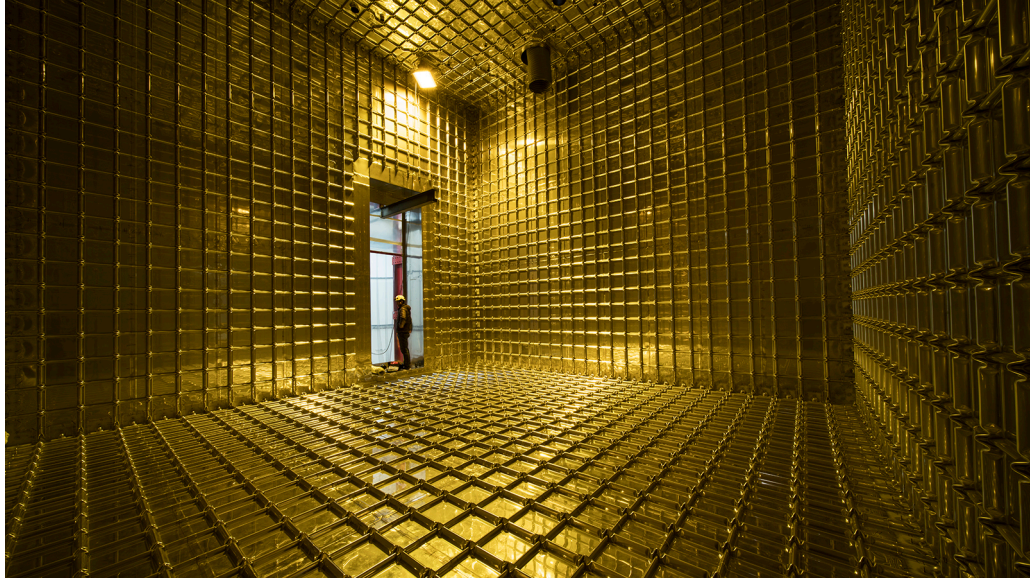
Figure 27: ProtoDUNE-SP membrane cryostat. Photo credit: CERN.
