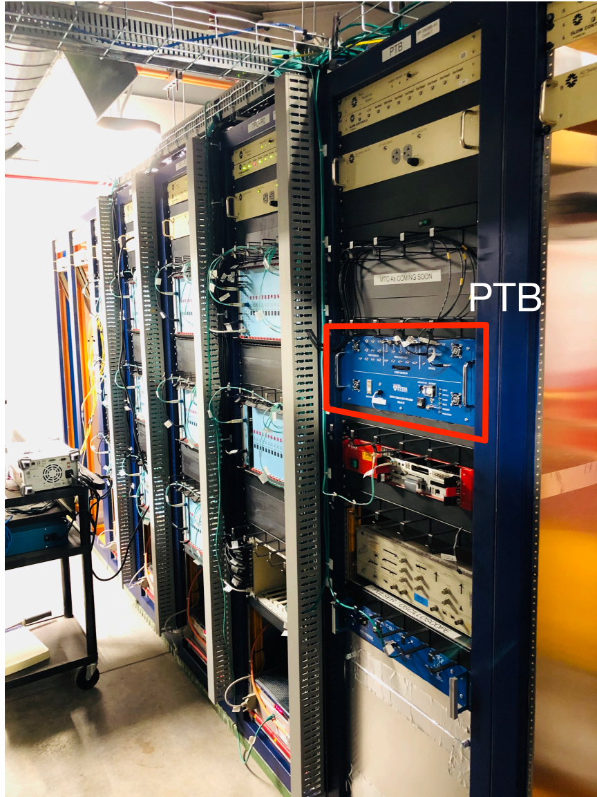
Figure 38: PTB at the Near Detector Building.
