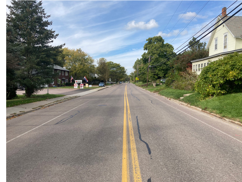
This image shows the 4' shoulder classified in the Transportation Master Plan as a bike lane.
