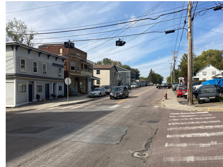
There are no intersection markings indicating a bike lane and the bike lane includes storm drains.
