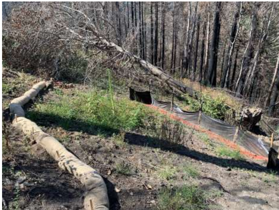
Figure 9. Downslope view of fully constructed silt fence plot and highlighting the red chalk.
