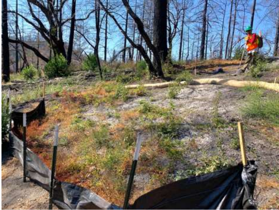
Figure 8. Upslope view of fully constructed silt fence plot.
