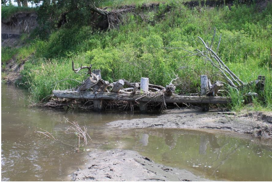
Figure S1. An example of a wooden jetty used on Cedar River as part of the 2005 Cedar River Stabilization Project.
