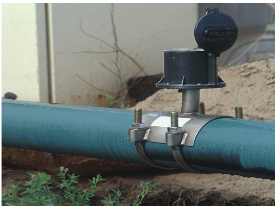
Figure 3.8. Field installation of a propeller meter.
