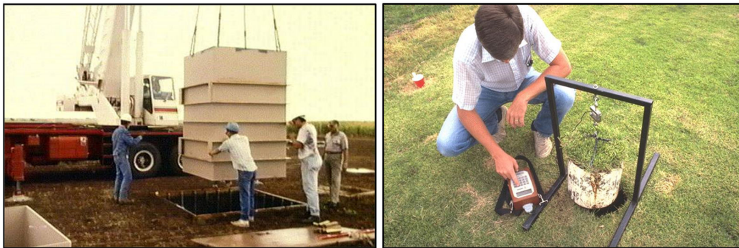
Installation of Large Precision-Weighing Lysimeter
