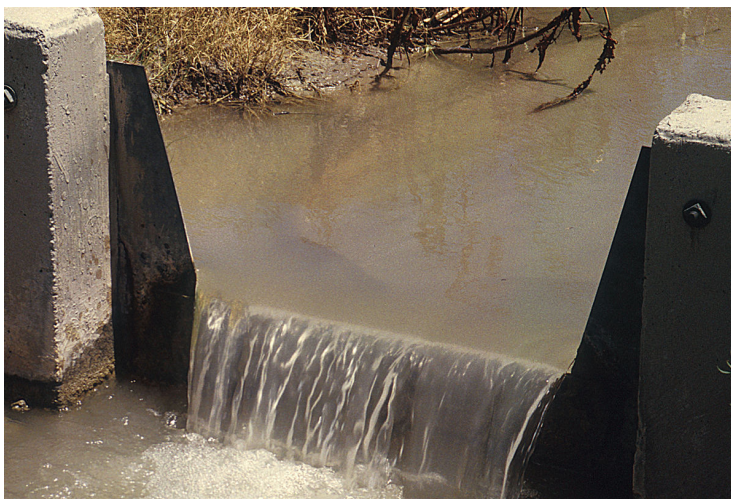
Figure 3.18. A weir for measuring water flow in an open channel.
