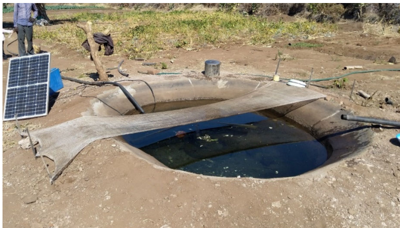
Figure 9.5. Water delivery system for groundwater from the shallow alluvial aquifer of the Shashe River, Zimbabwe. A solar pump is used to deliver water from the concrete-lined storage pond to a nearby field, and the net provides shade for fish. (Photo courtesy of Annelieke Duker, IHE Delft Institute for Water Education.)
