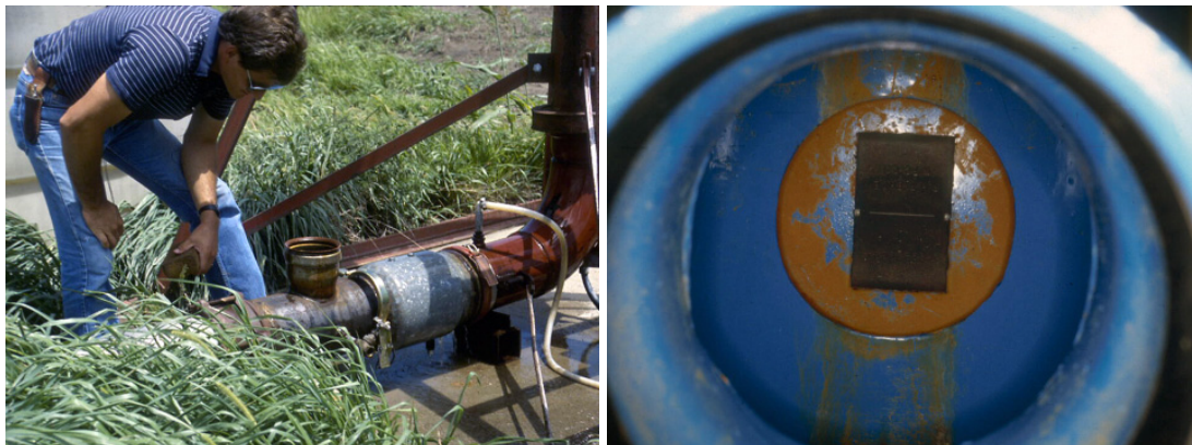
Figure 15.7. Inspection for check valve leakage in CCVA.
