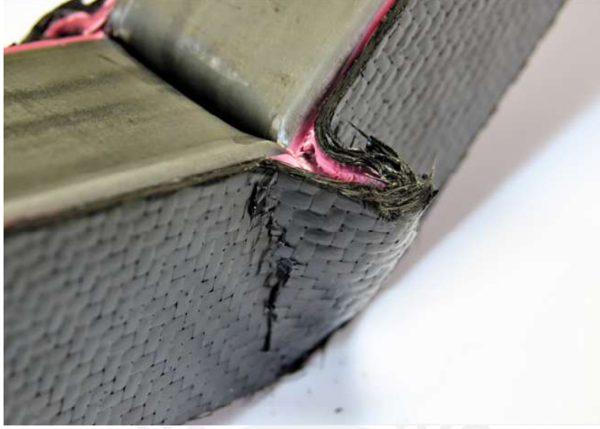
Figure 5.18: Collapse zone that forms in LR50x2, note that the fracture grows from the upper part to the bottom.
