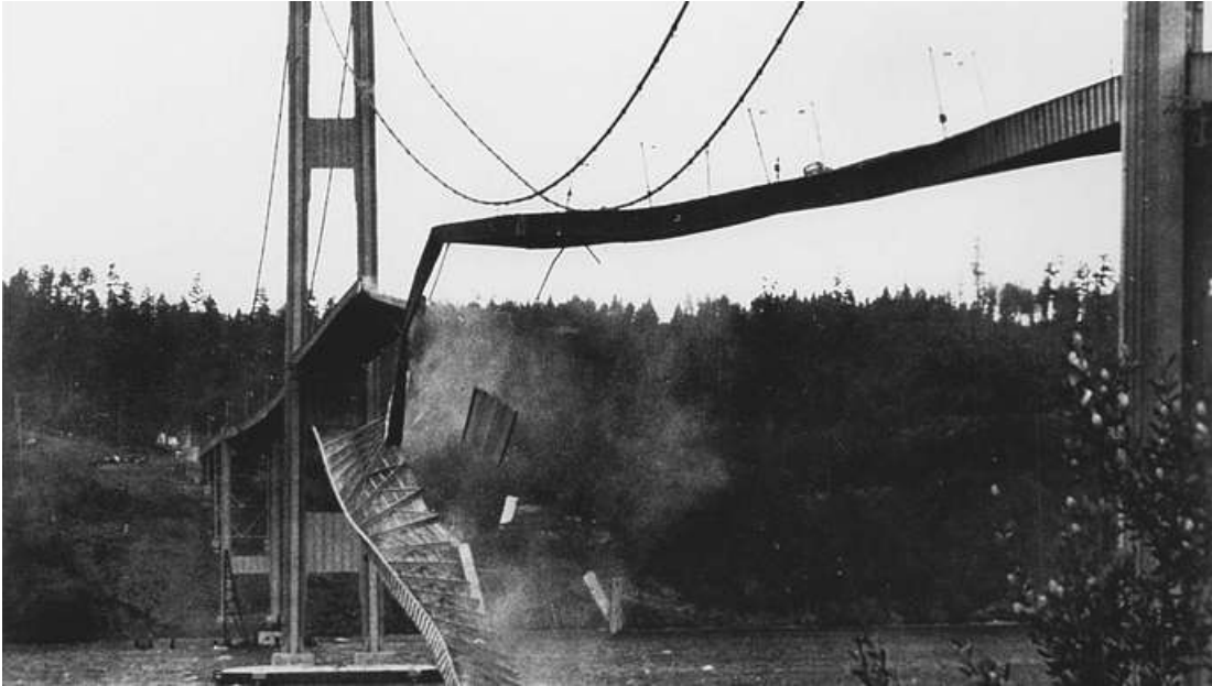
Figure 3.1: Tacoma Narrows bridge after having collapsed; source https://www.britannica.com/technology/bridge-engineering/Tacoma-Narrows .
