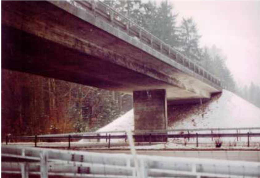
Figure 3.2: Photo of the Z24 bridge.
