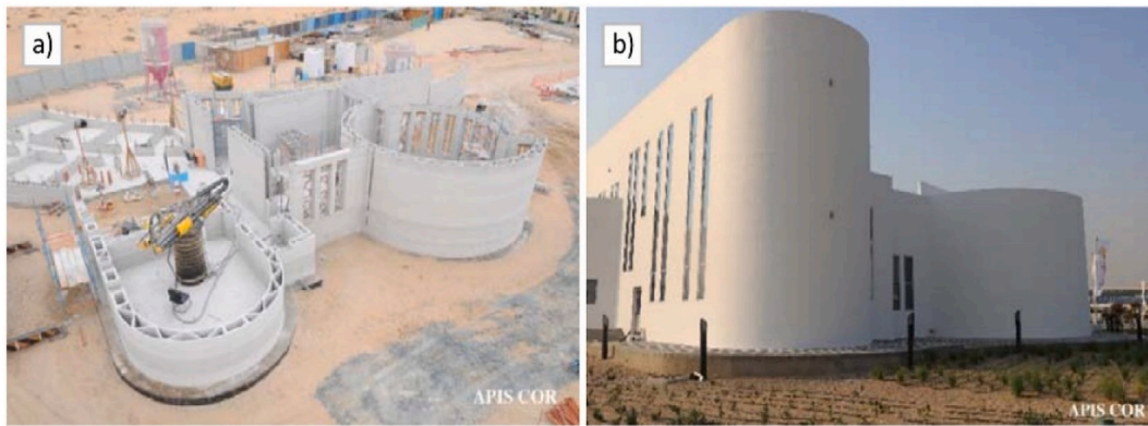
Fig. 12. (a) Printing stage and (b) complete view of the world's largest 3D printed house by Apis Cor in Dubai [21,201].
