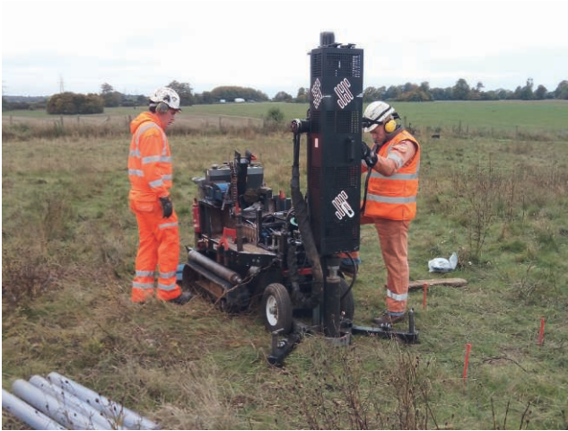
Figure 2. Coring rig on site.
