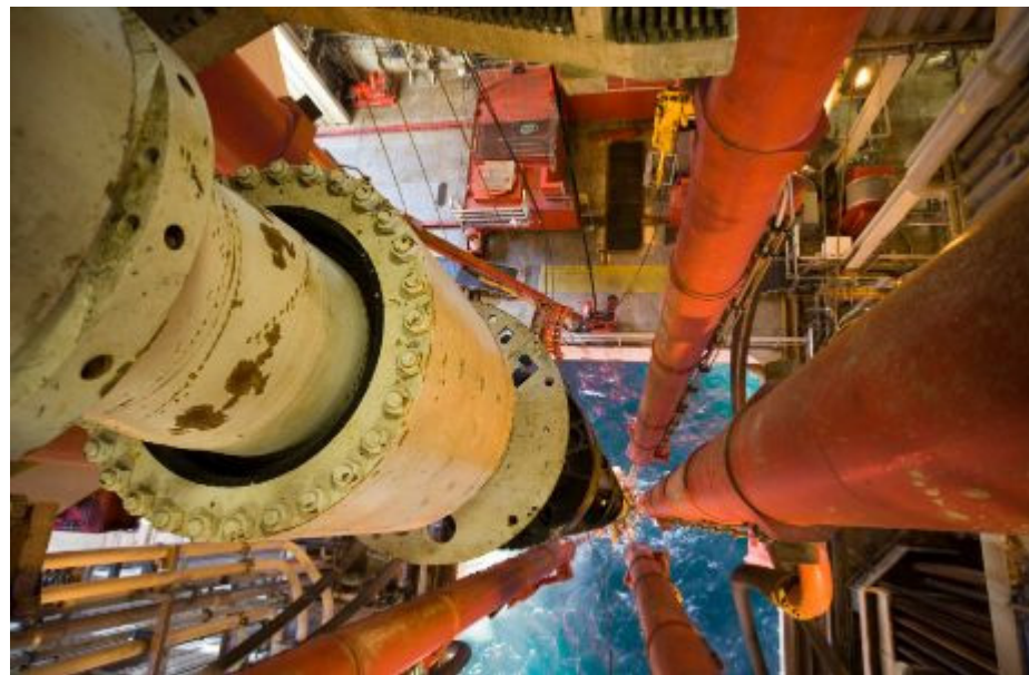
Figure 2. An aging offshore platform showing the marine riser.
