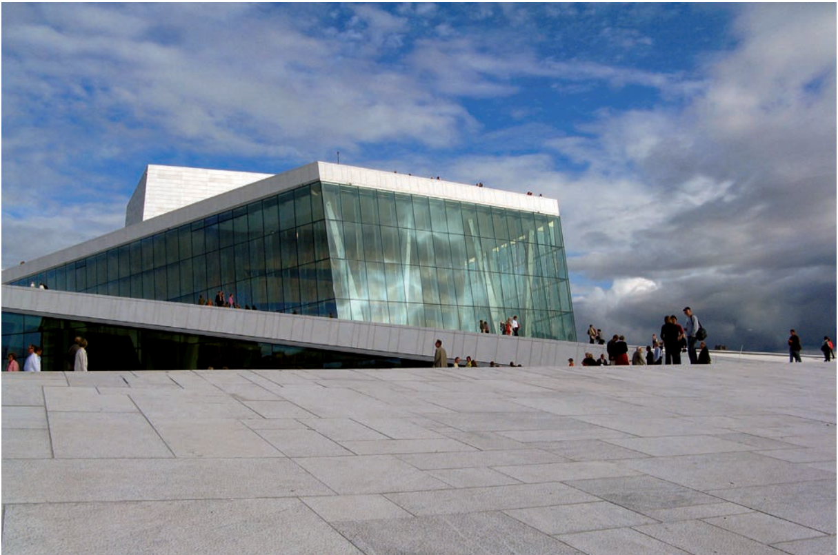
Figure 4.2: Oslo opera house (2008) built from Italian Carrara marble. Photo courtesy Tom Heldal; source: EuroLithos-project.
