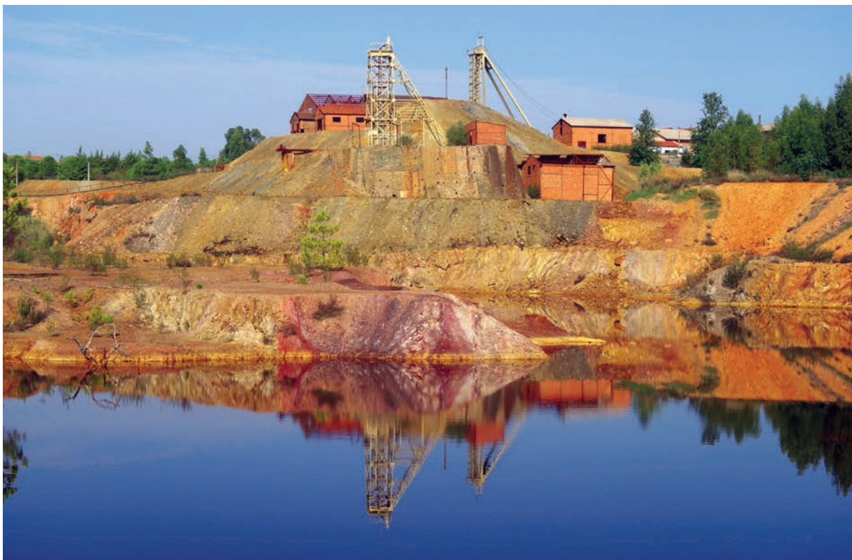
Figure 2.13: View of the Lousal open pit (foreground) and the mine dumps, headgears and ore processing plant in the background. Photo courtesy of Daniel de Oliveira.
