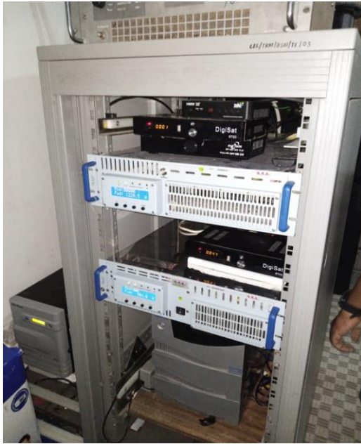
Figure 38: Broadcasting transmitter within the equipment room
