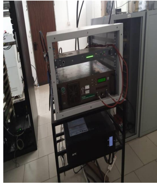
Figure 38: Broadcasting transmitter within the equipment room
