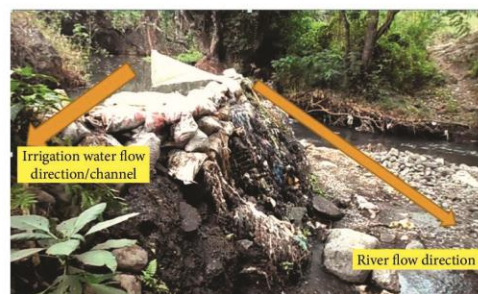
FIGURE 5: Furrow intake constructed with sand bag/stone/trees logs.
