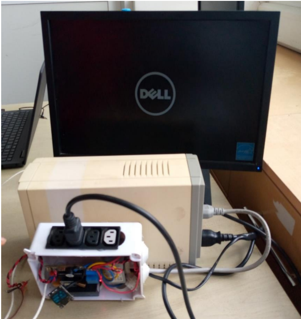
Figure 32: Main System Connected to the UPS and the load During Testing
