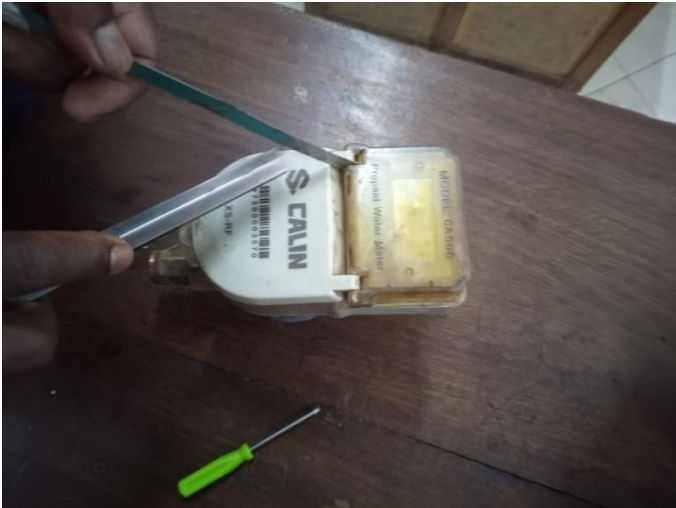
Figure 6: Opening a prepaid meter before removing a top cover
