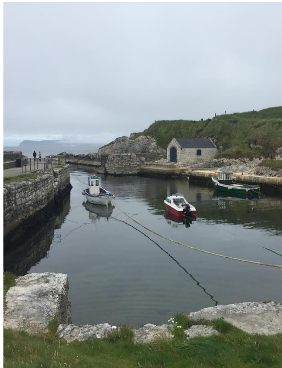
Figure 6.9: Photo of Ballintoy Harbour
