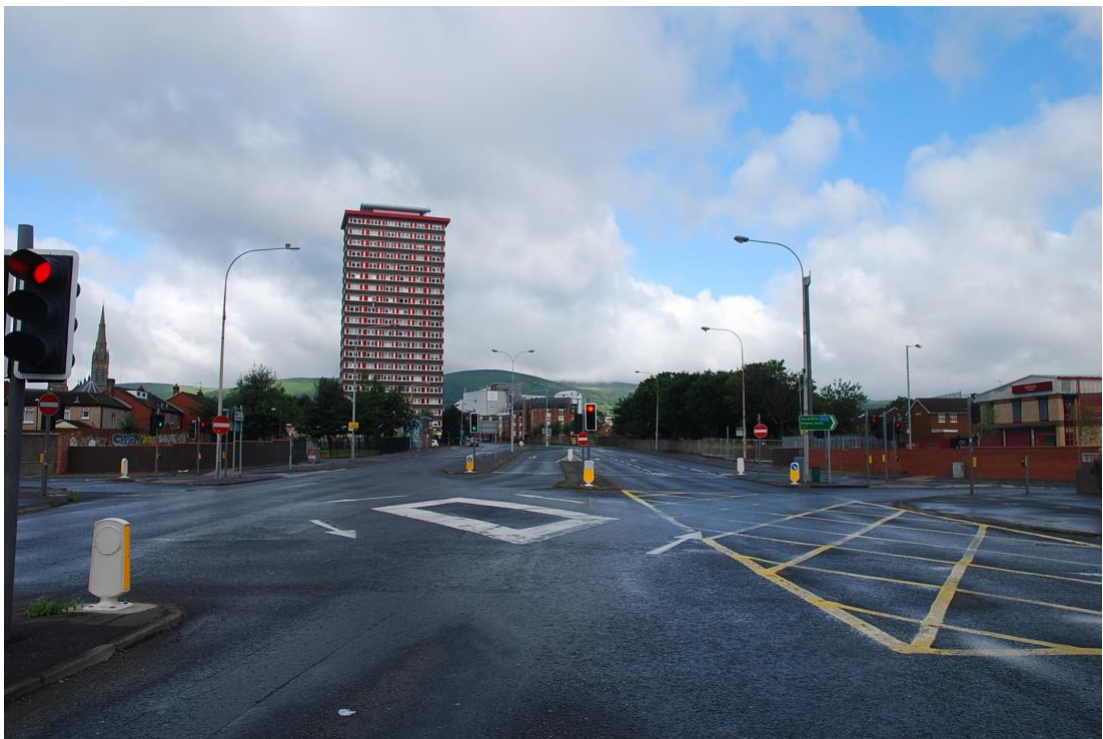
Divis street junction with the Westlink Motorway. From the late 1960s until the late 1990s the British Army had an observation post located at the top of the tower. Photograph by Tim Cunningham, July 2015
