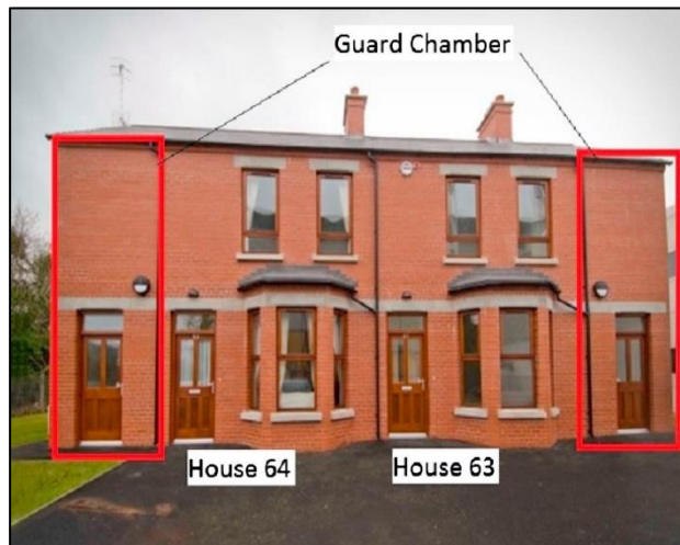
Figure 3 - Test Houses at Ulster University, Jordanstown Campus [36]. The electricity consumption of house 64 was used for the present study.
