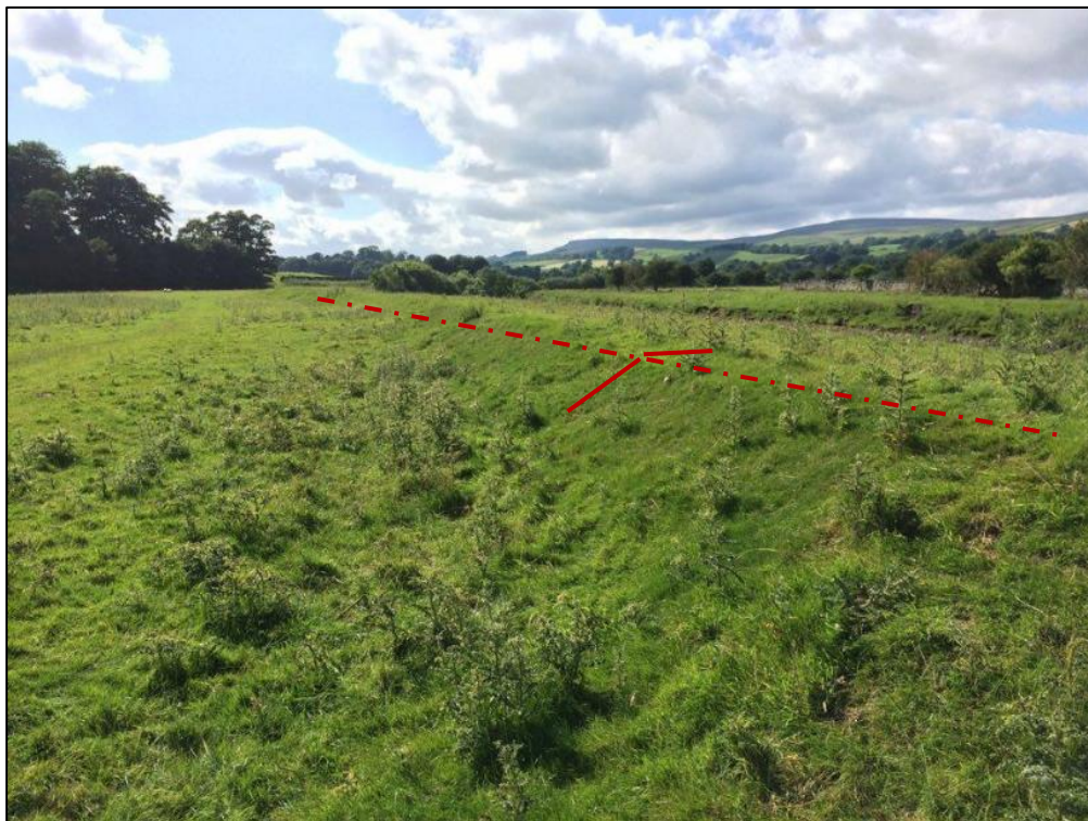
Figure 4-13 Photograph showing a length of embankment alongside reach PR006, as observed during field data collection
