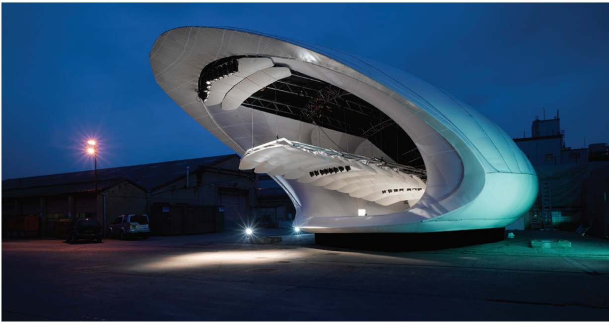
Fig 5.4.13 The acoustic panels being lifted into place during the test in London's docklands.
