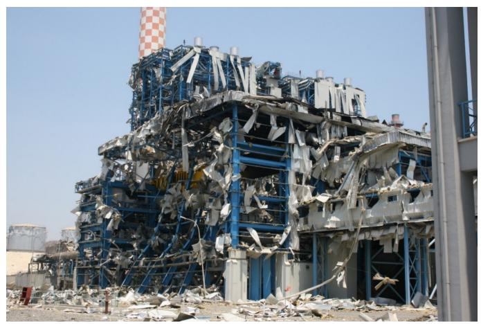
Figure 3. Vasilikos power station after the Florakis Naval Base explosion, Cyprus. Source: photo courtesy IDE Technologies Ltd.
