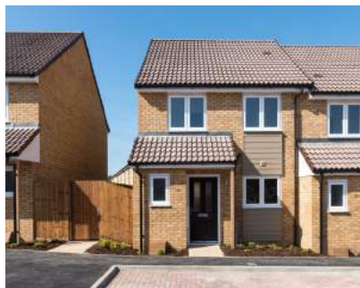
Paradigm's design & build site at Caleb Close in Luton. Caleb will deliver 224 affordable homes with a mix of rent, shared ownership and outright sale.
