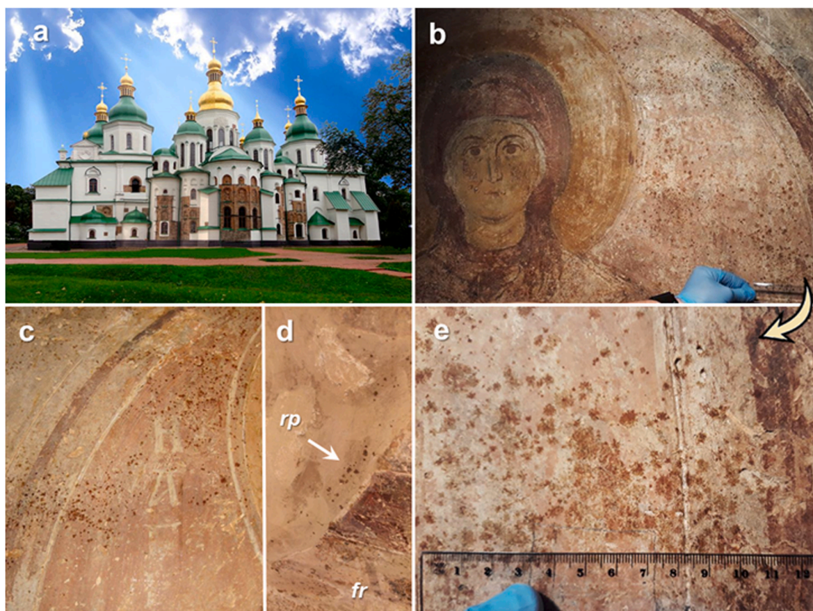
Fig. 1. (a) A current view of St. Sophia's Cathedral, 11th c., Kyiv, Ukraine; (b–e) dark spot deterioration on the medieval frescoes on the cathedral walls; (d) spread of dark spots on areas of the frescoes (fr) and restoration plaster (rp) shown with white arrow; (e) a detailed view of the right, bottom corner of (b).
