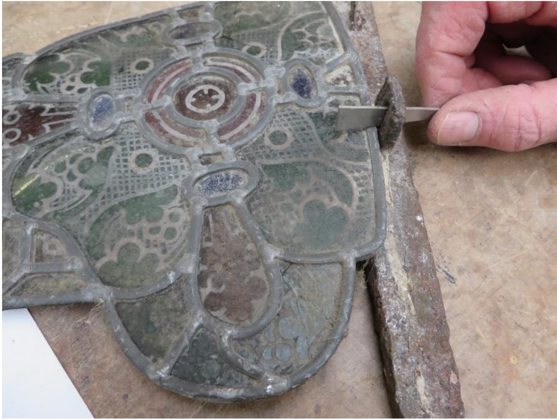
Figure 7: Leaded glass, glazing bar, eye, and wedge
