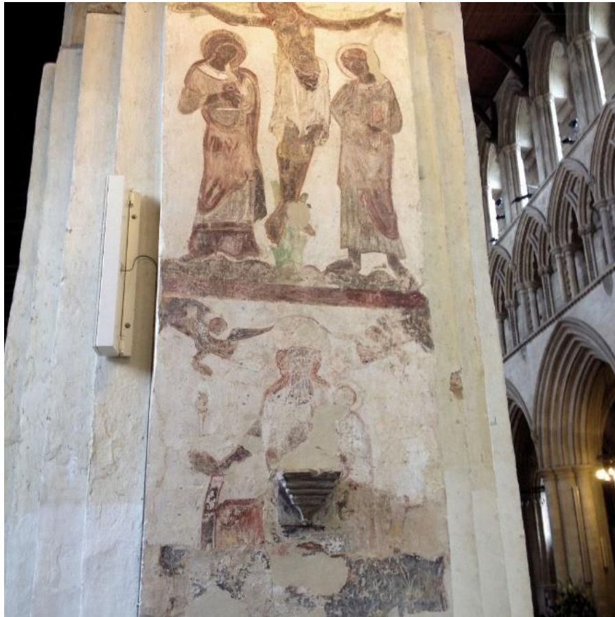
Figure 3-28: St Alban's Cathedral - plinth inserted in lower painting for support of light
