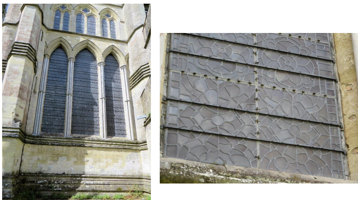
Figure 3-8: South-east vestry window showing ferramenta
