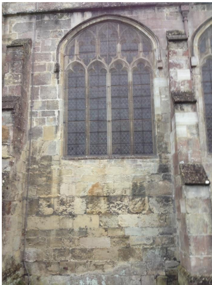
Figure 5-2: Window of four major lights at St Edmund's on the south side of the chancel
