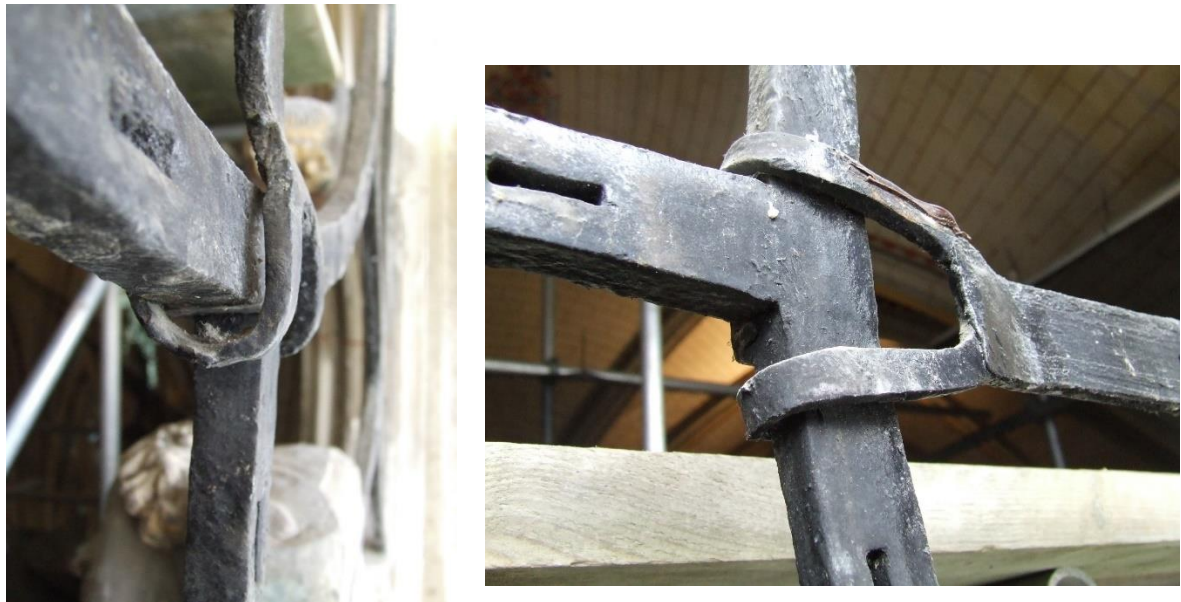
Figure 6: Close-ups of metal work at Salisbury Cathedral
