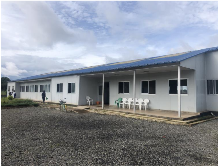
Figure 2-2. External façade of the 'Ebola Camp' in Mzuzu Photo taken by Alexandra Viner.
