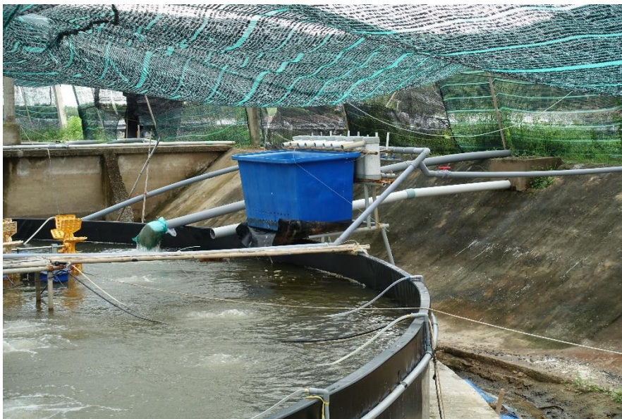
Figure 36 A protein skimmer for a super-intensive shrimp pond
