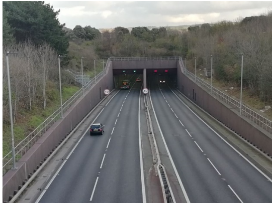
Figure 15: Photo of the western entrance of the Conwy Tunnel. 821
