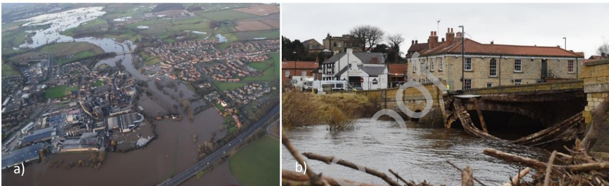
Fig. (4): Tadcaster 2015 flood from Storm Frank where (a) Shows aerial imagery of the flood affected zone (source: Environment Agency), and (b) highlights an example of the extent of the damaged infrastructure (source: BBC, 2016)
