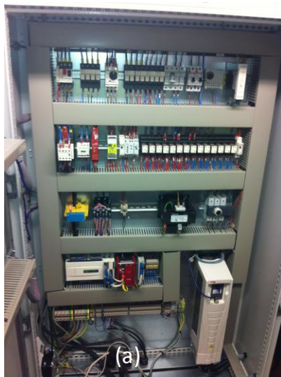
Figure 46. Data monitoring and acquisition unit.
