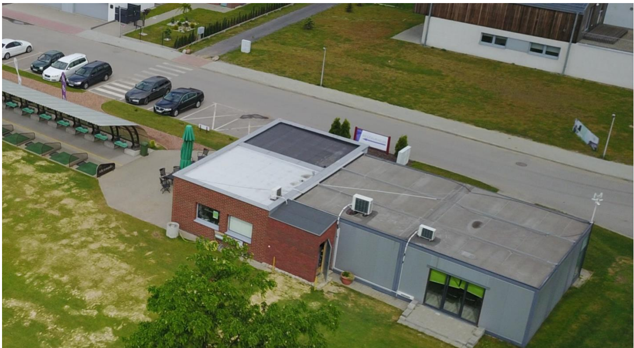
Figure 64. Final look over installation container
