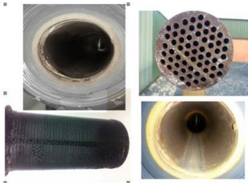
Figure 19 Inspection of pipelines at Markham
