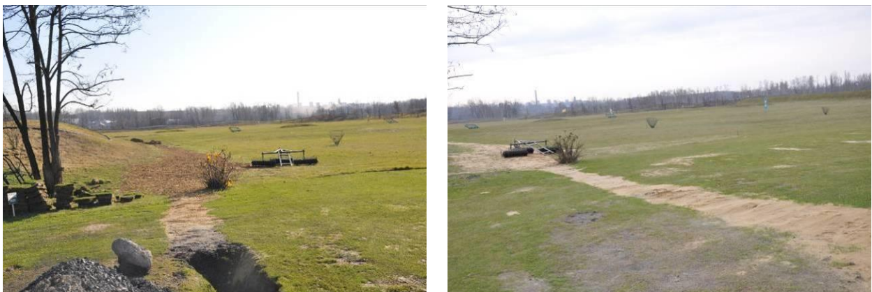
Figure 62. Excavation for a pipeline (connection between buffer tank and container).
