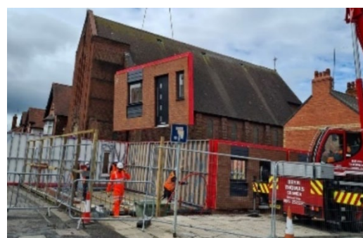
Figure 4. MMC - assembly of building elements at site (Starship Group, 2021)
