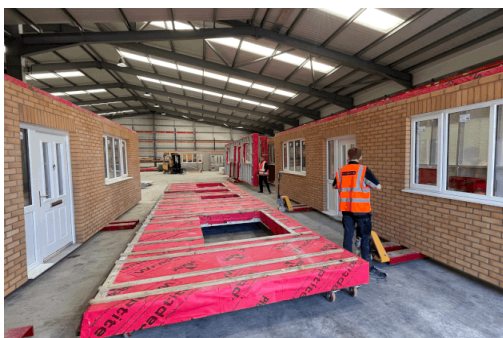
Figure 3. Offsite manufacture at Deeside factory (Starship Group, 2021)
