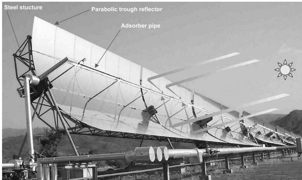
Figure 2.10: Parabolic trough collector [7].
