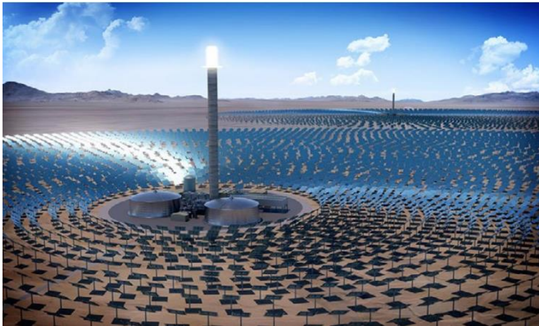
Figure 2.11: Central receiver tower [70].
