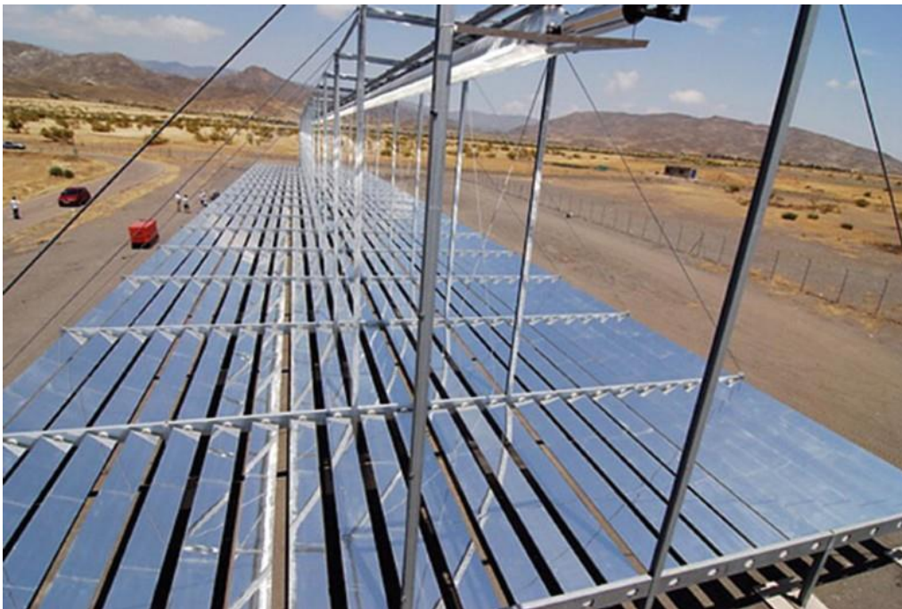
Figure 2.12: linear Fresnel reflector (LFR) [80].
