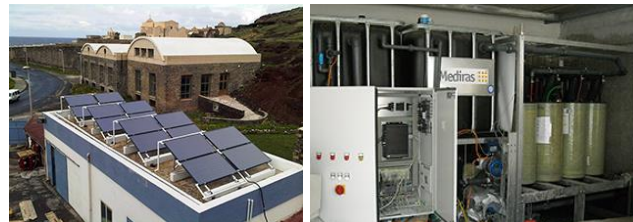
Fig.1: Multi module two loop system in Pantelleria, Italy. On the left: solar thermal collectors; on the right: membrane distillation modules.
