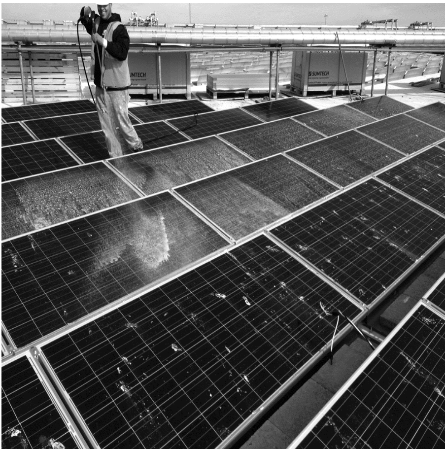
Figure 2. Researchers found that dirty solar panels only lose about 7.4 percent of their efficiency.
