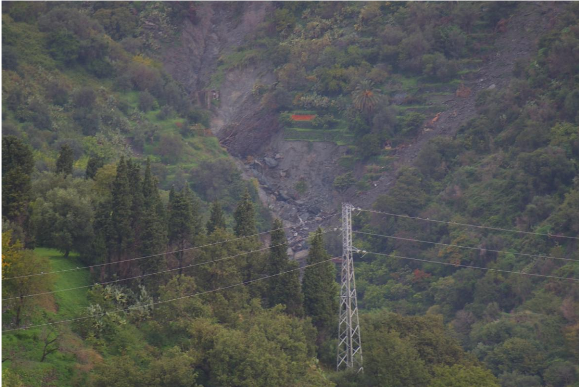
Figure 4.2 - Material transported across the slope to intersect the river network.
