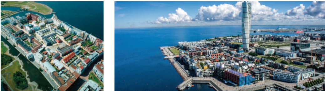
Figg. 43, 44 - L'eco-quartiere Bo01 - City of Tomorrow (1998-2001) a Malmö, © Bo01.
