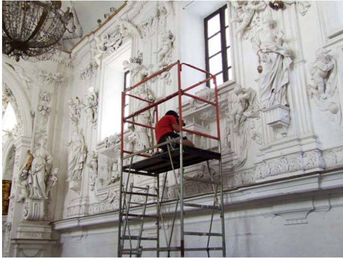
Figure 5: Oratory of St. Lawrence, Palermo. The photogrammetric survey campaign has been conducted with the assistance of a rolling scaffold, which allowed to reach the height of 4.40 m of planking level, assuring a correct frames shooting.
