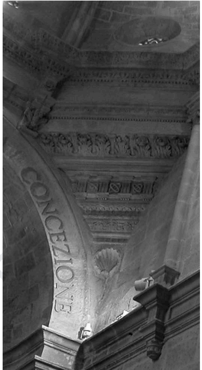
FIG. 17. Detail of a pendentive of the dome of chapel Naselli in the church of San Francesco in Comiso (Sicily).
