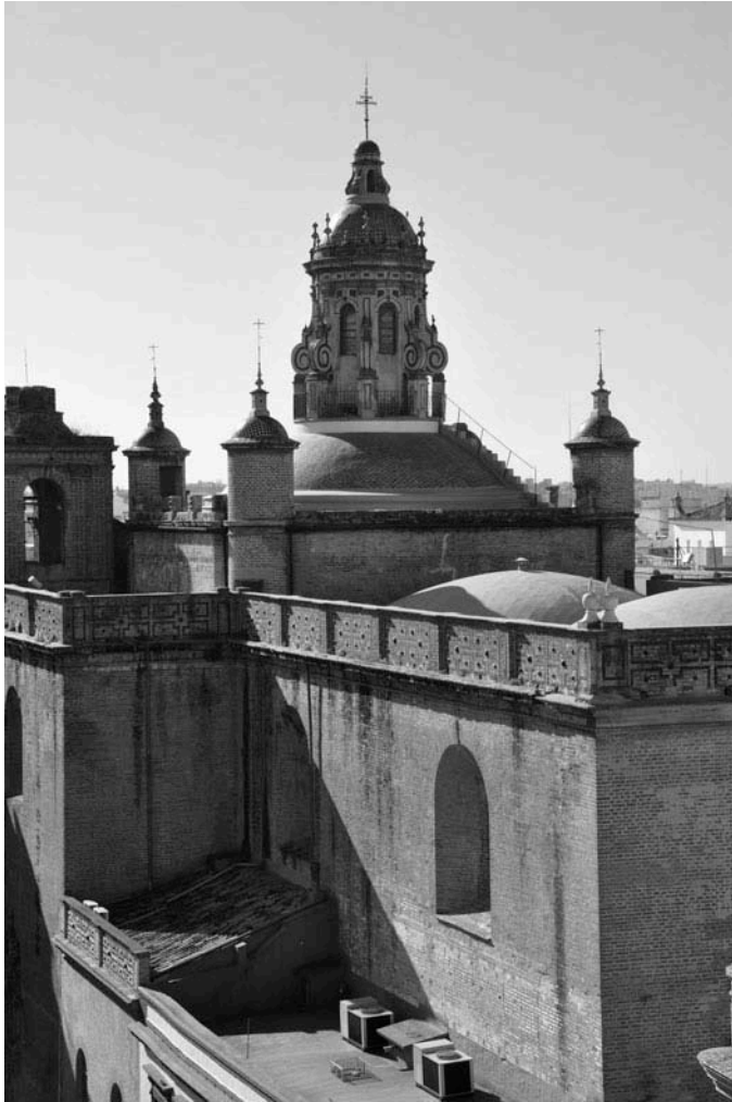
FIG. 18. View of the half-tiburium of the church of the Jesuit Professed House dedicated to the Annunciation in Seville.
