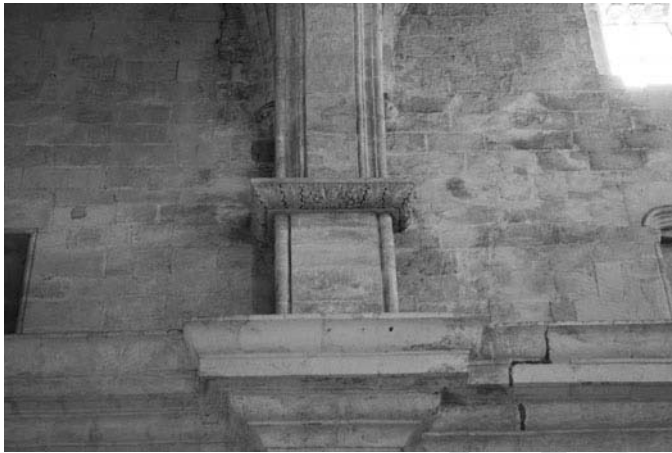
FIG. 7. Detail of the low-order of pilasters defined more gotico above the cornice in the Jesuit church in Sassari (photo by author, authorization of the Archdiocese of Sassari). © [rightsholder]. Reproduced by permission of [rightsholder]. Permission to reuse must be obtained from the rightsholder.
