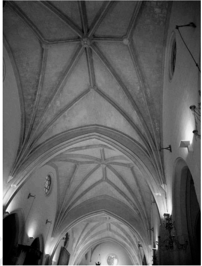
FIG. 2. Sequence of vaults with five keystone on the nave in the church of S. Eulalia in Cagliari (photo by author).
