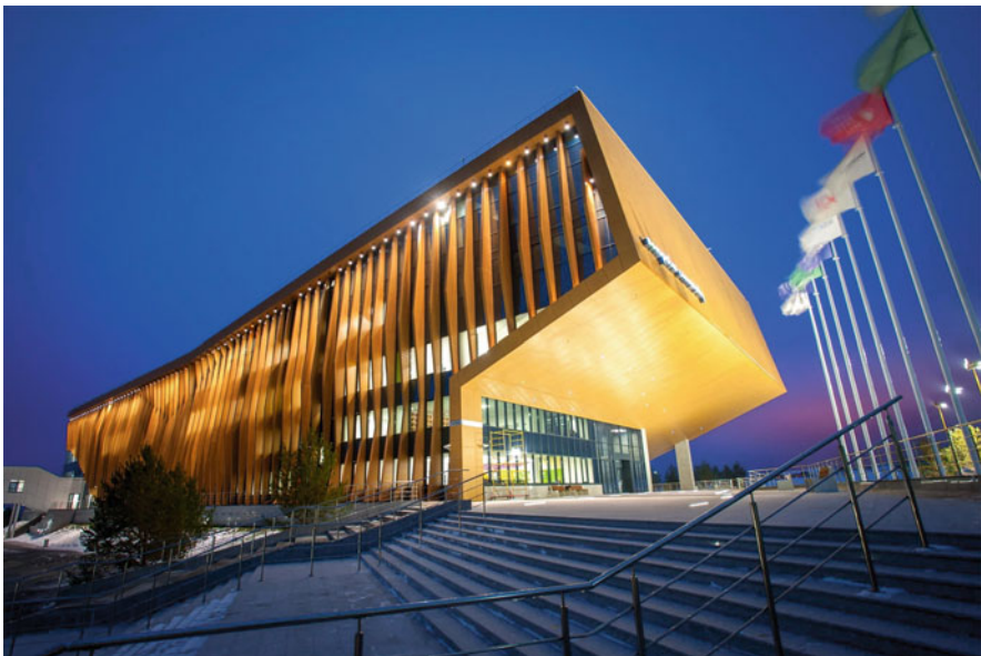
Fig. 2.2 The university building
