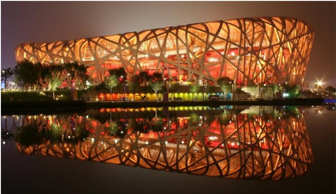
Fig. 27-28. The Olympic stadium in Beijing by Herzog & De Meuron
