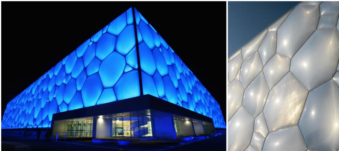
Fig. 28-29. The watercube by PTW Architects in Beijing.
