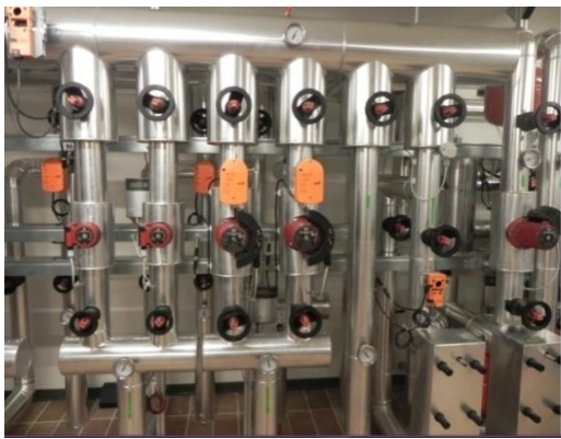
Figure 21 electropumps and electrovalves operation on the collectors system
