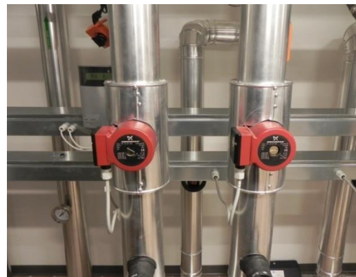
Figure 21 electropumps and electrovalves operation on the collectors system
