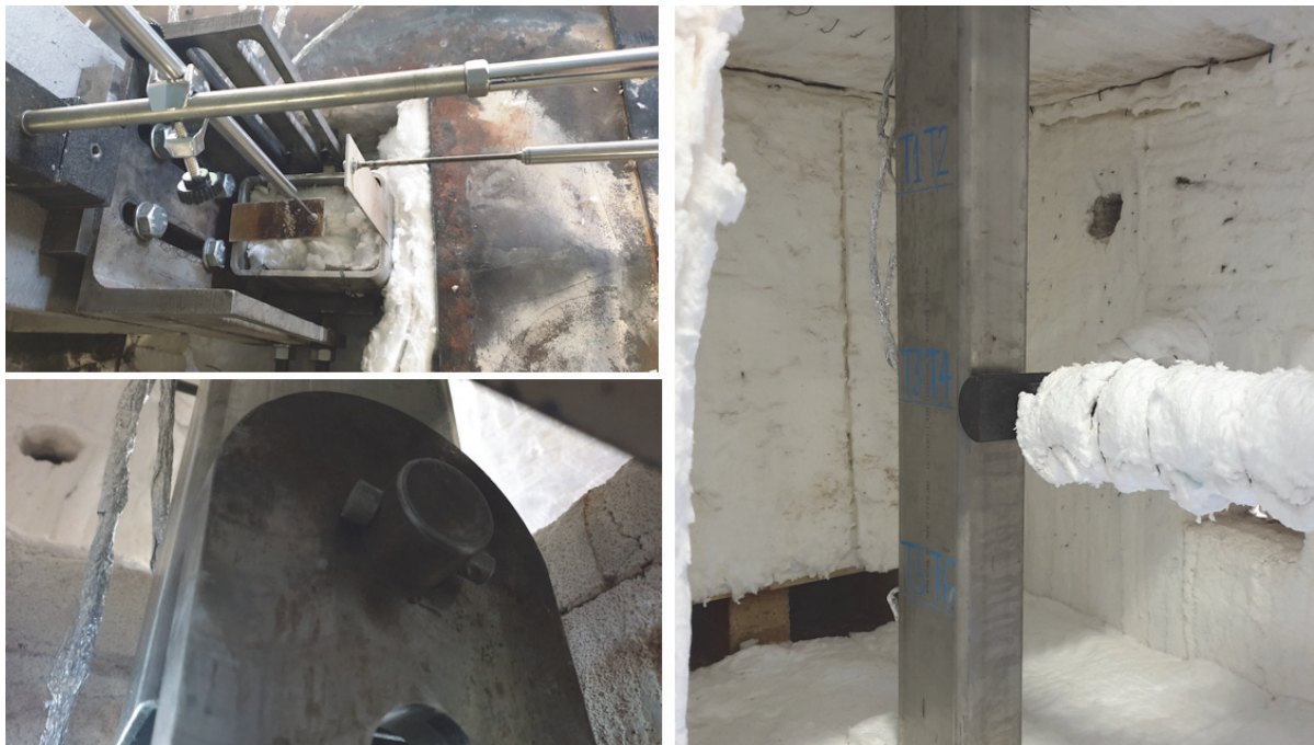
Fig. 2 – Beam inside the furnace and supporting conditions.
