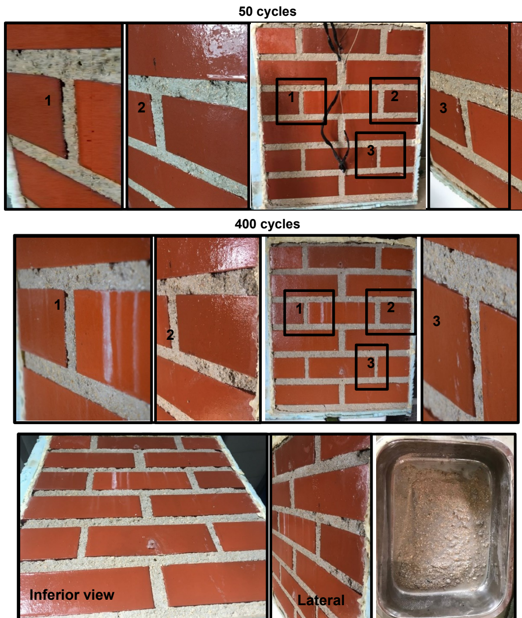
Fig. 9 – Visual aspect of the brick veneer wallets after freeze and thaw cycles
