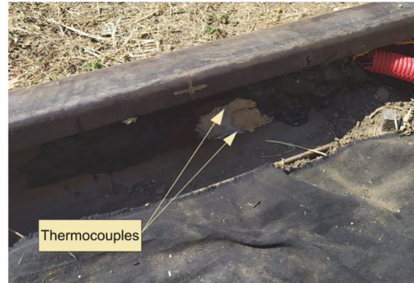
Fig. 4 – Installation of thermocouples.
