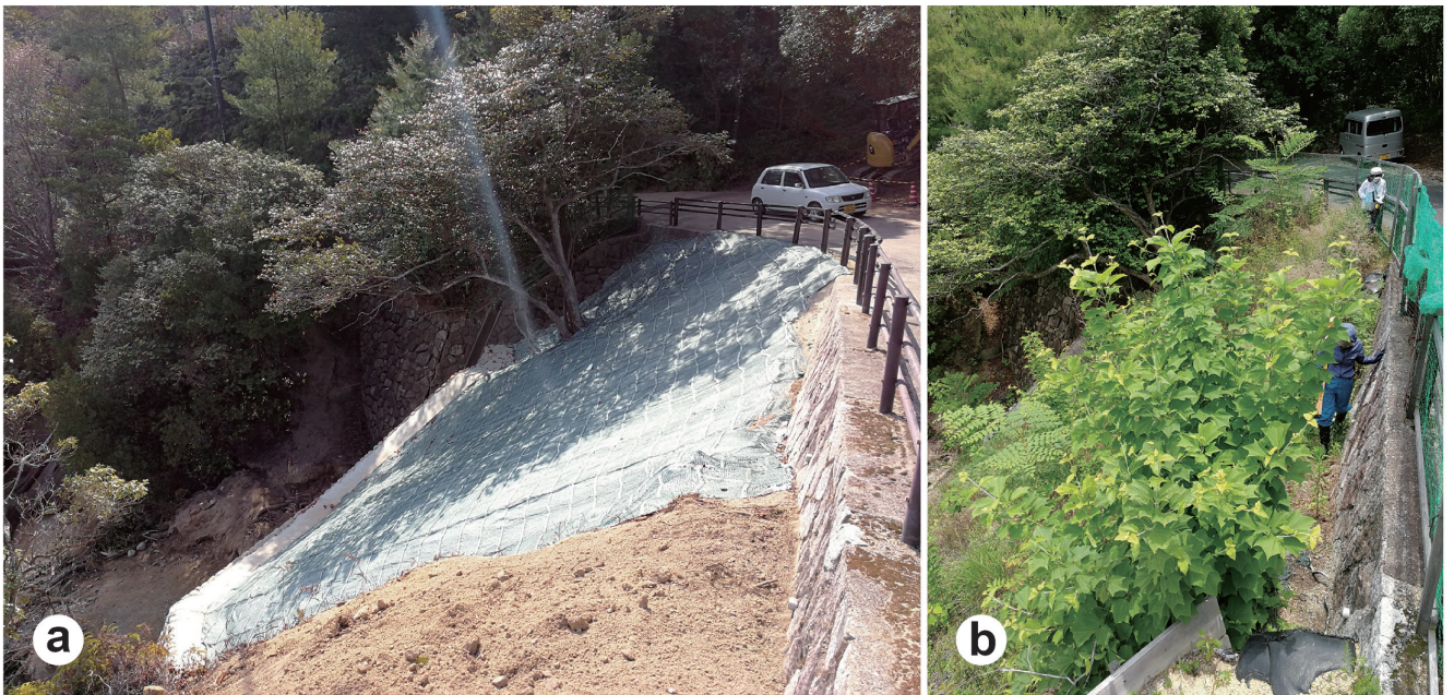
図1 大元一多々良地区の土砂災害跡地の緑化工前 (a; 2019年4月) と緑化工後約2年後 (b; 2021年6月) の様子 Fig. 1. Before (a) and after (b) revegetation work in Ohmoto Park-Tatara restored site, Miyajima Island, Hiroshima Prefecture, Japan, April 2019 (a) and June 2021 (b). The community after two years includes young trees ( Acer rufinerve , Quercus glauca , Aralia elata , etc.), and high herbs and grasses ( Artemisia indica var. maximowiczii , Miscanthus sinensis , Perilla hirtella , etc.). Photos by H. Tsubota.
