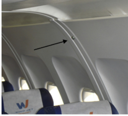
Fig. 3. Position of a temperature/humidity sensor in the wall of the cabin.
