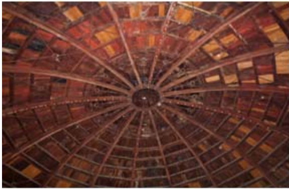
Figure 2 - Interior view of the dome
