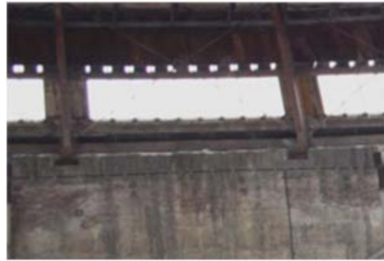
Figure 3 - Connection between ribbings and curb
