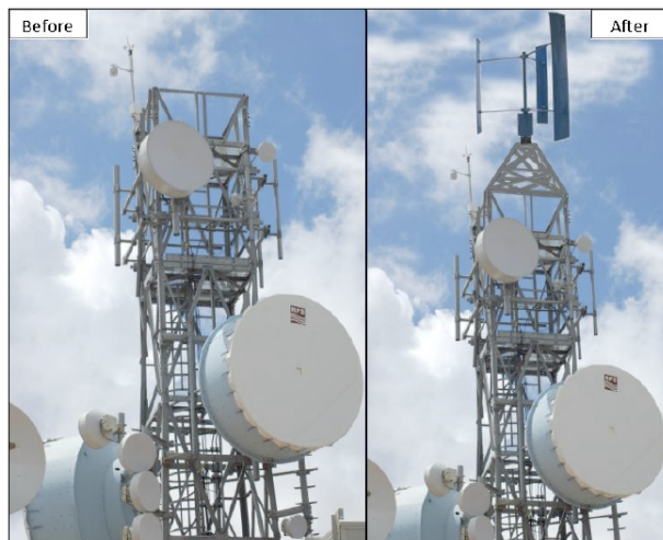
Fig. (8). Tower before and after vertical axis turbine installation.
