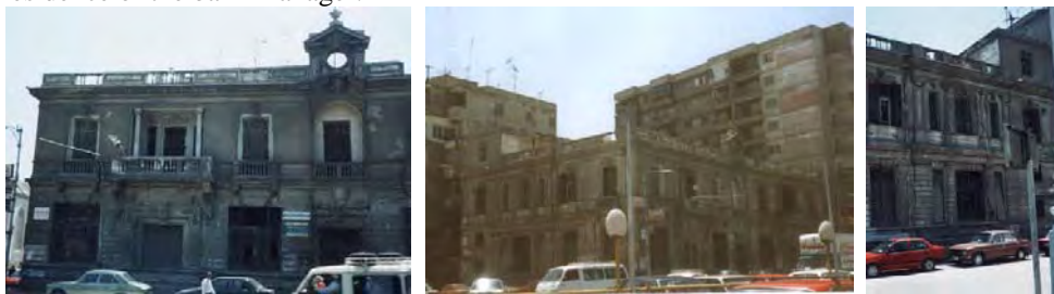
Fig.11. Bank of Alexandria before restoration.
