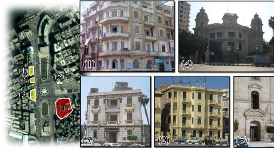
Fig.17. El-Geash Street& Om-Kouthom square. (1),(2),(3).private residential and office buildings, (4). palace now the Police headquarter, (5).residential building in ruins.
