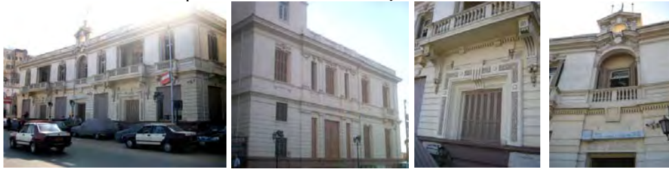
Fig.12. Façades and details of “Bank of Alexandria” after restoration.
