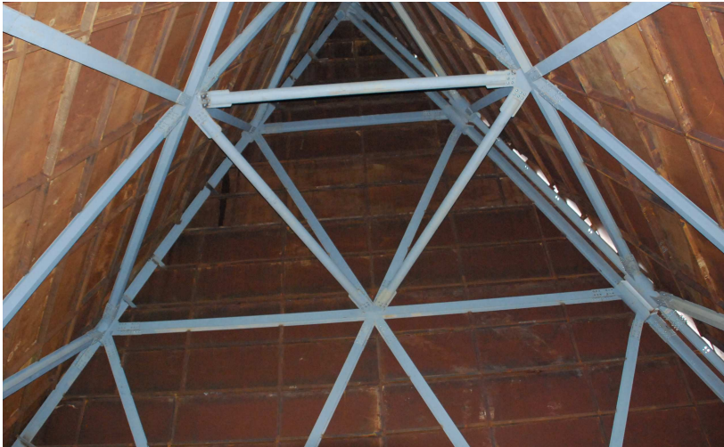
Figure 8: Inside view. Framed alveolar steel structure.
