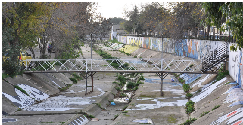
Fig. 1: The old bridge to be dismantled
